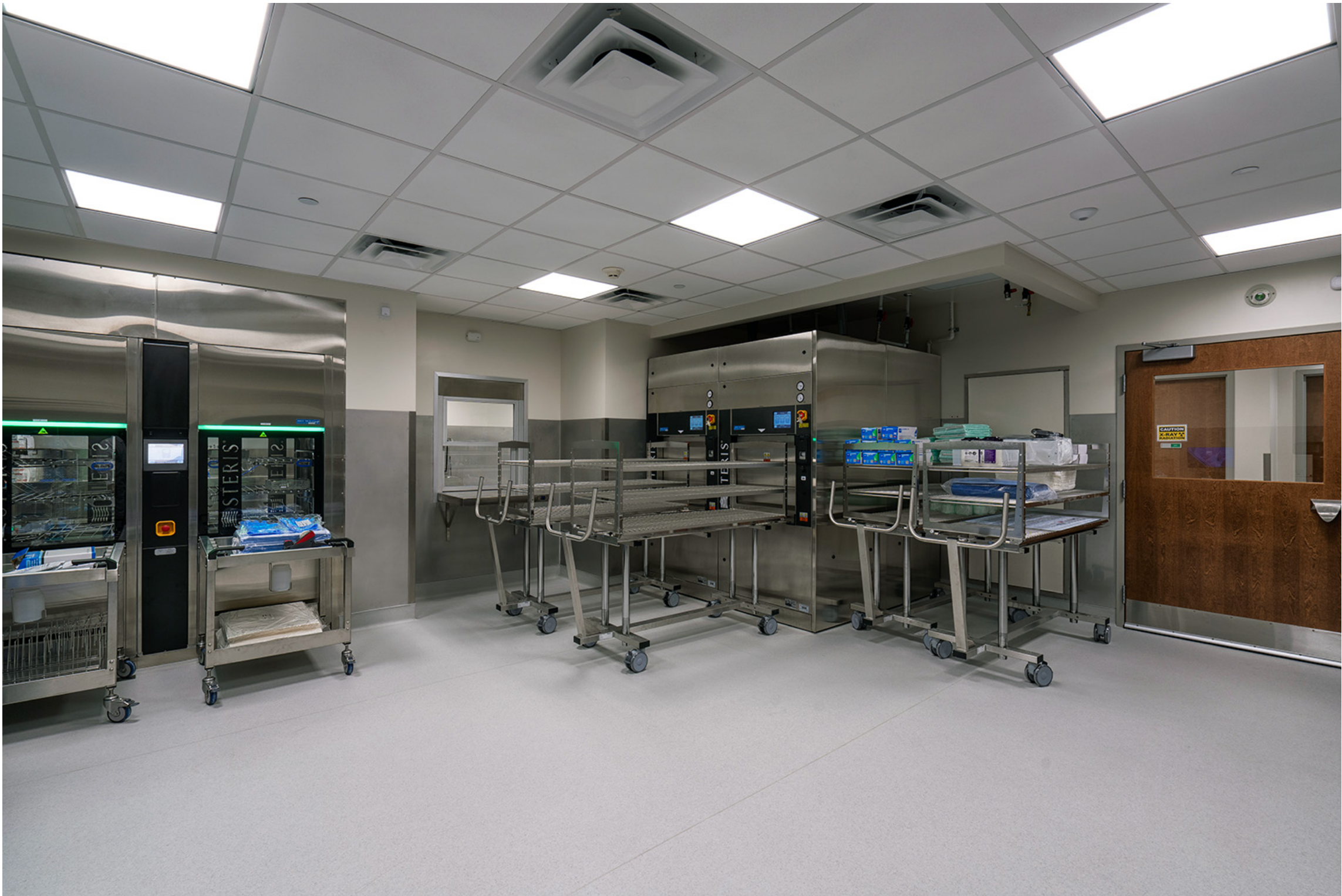
Sterile processing | Completed interior
